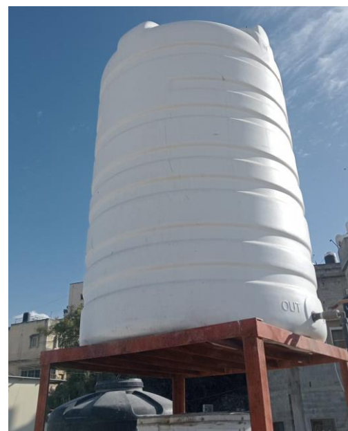
A distributed water tank has installed on the roof of one of the beneficiaries.
