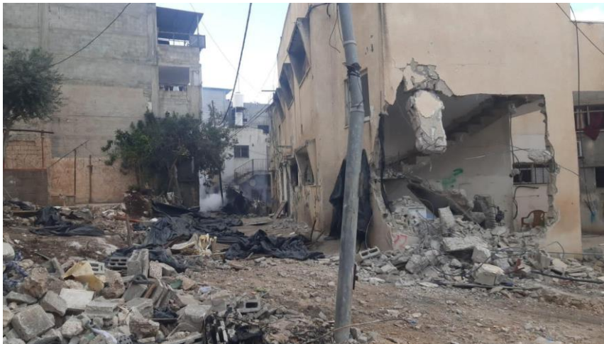
(Damaged infrastructures of Nur Shams Refugee Camp)
